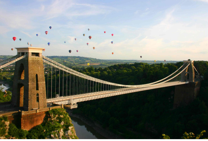
Figure 24.1: Clifton suspension bridge, Bristol, UK. The cables of a suspension bridge hang in a shape which is almost (but not exactly) a parabola.
